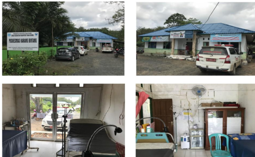
Fig. 1. Health center Non Care Karang Bintang and ER Health center Non Care Karang Bintang, Health Office Tanah Bumbu District, South Kalimantan Province
